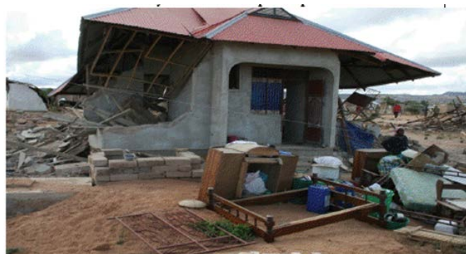
Plate 1: A house involved in demolition in Njedengwa at Dodoma-Makulu Ward (2011)
